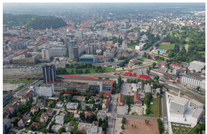
FIGURE: COMMERCIAL, PRODUCTION, AND WAREHOUSE SPACE LIKOZARJEVA IN LJUBLJANA
